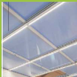
Illuminazione a LED LED lighting
